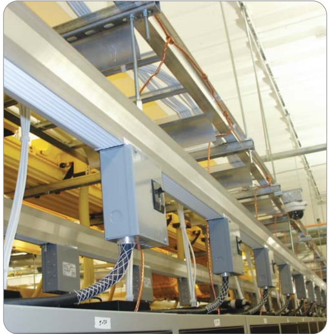
Power can be accessed at any location along the busway system, eliminating the need for power boards, long runs of wire and expensive installation costs.
